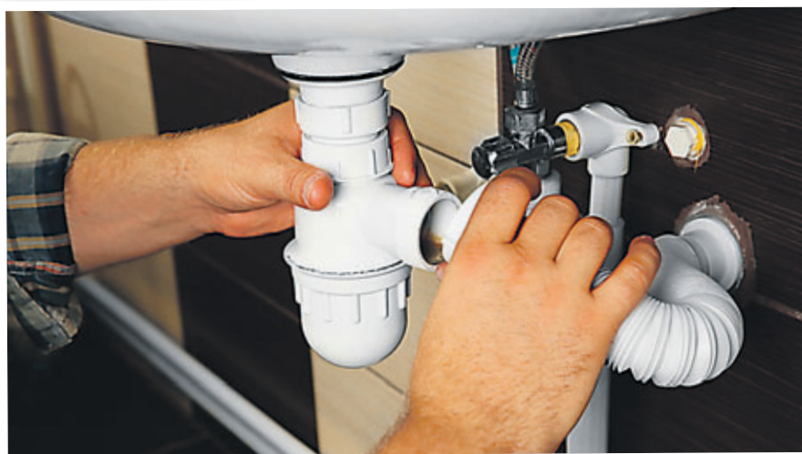
CLOGGED DRAINS: Right Plumber offers drain cleaning to tackle the toughest clogs.
