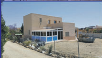
FINISHED GLASS ENCLOSURE WITH TILED EFFECT ROOF AND BRONZE TINTED GLASS
