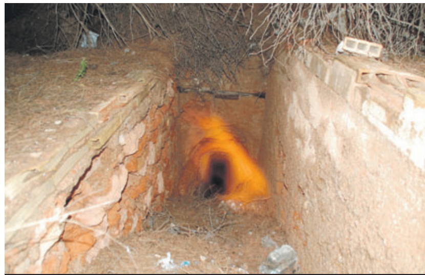
MYSTERY STRUCTURE: Gradient leads to what appears to be a tunnel.
