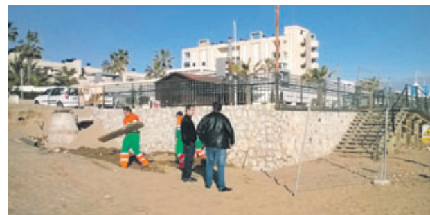
PROMENADE WORK: Repairs underway in La Mata.
