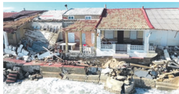
PLAYA BABILONIA: Collapsed and damaged houses.
