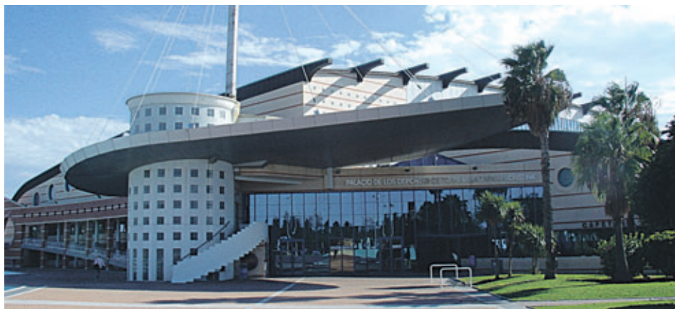
REPAIR WORKS: Include improvements to the changing rooms.
