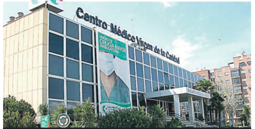
CENTRE EXPANSION: Will house 38 individual rooms and a cafeteria.
