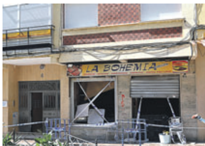
BLAST: Occurred in the bar's kitchen.
