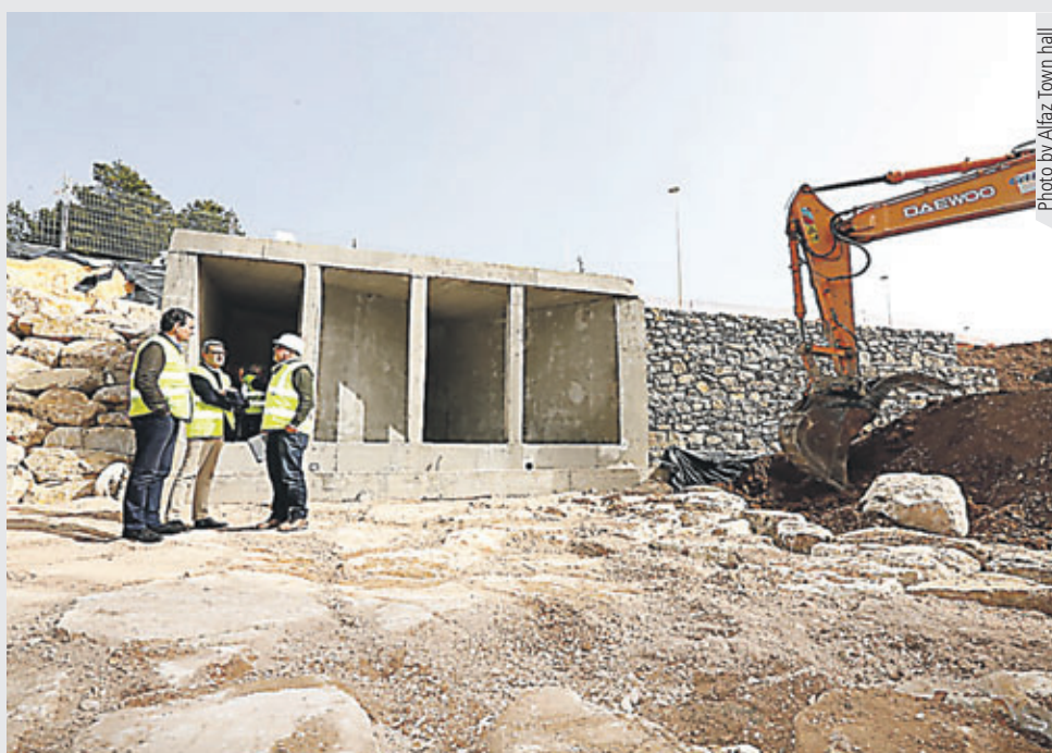
NEW OUTLET: Will slow down the water before it enters the Barranco de Soler stream.
