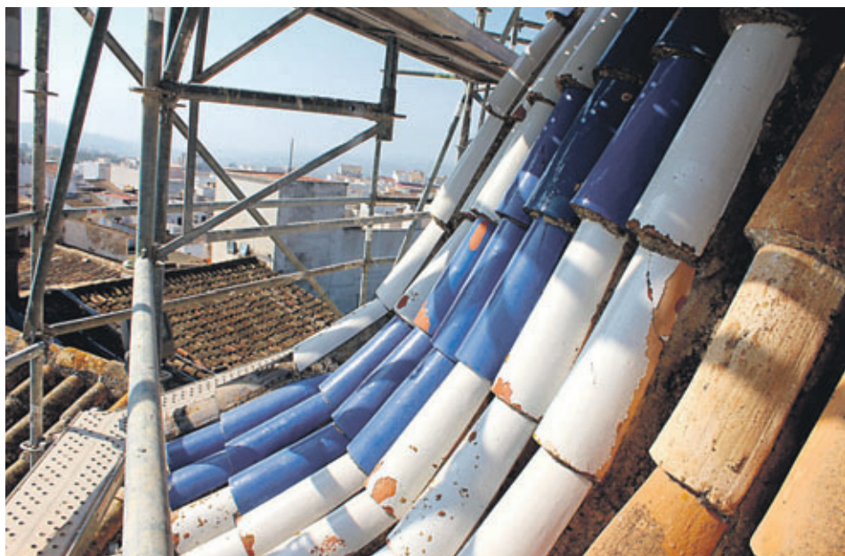
DOMES REPAIRS: Reproducing the original blue and white pattern.
