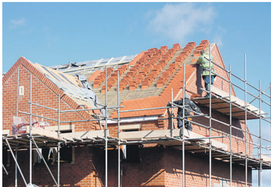
NEW HOMES: Found to have problems with infrastructure and construction.
