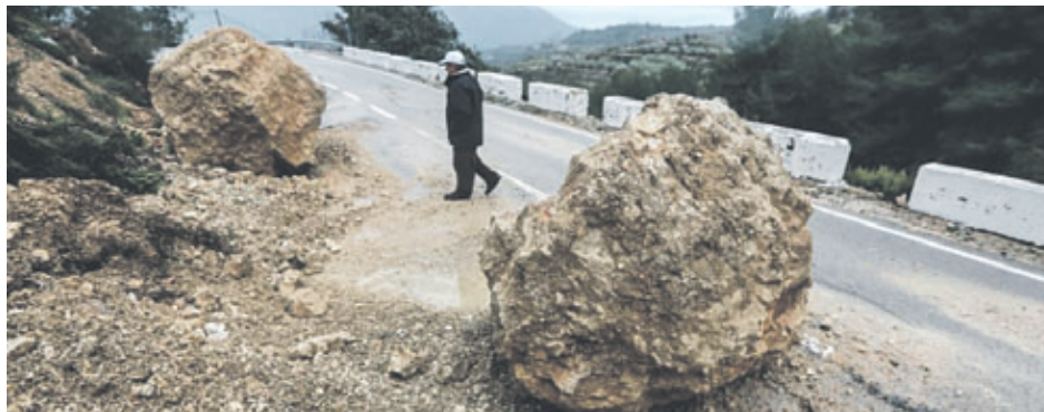
STORM DAMAGE: Giant boulders lie on the CV-70.
