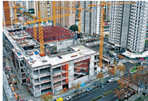
RESUME WORK: On the Benidorm Culture Centre.
