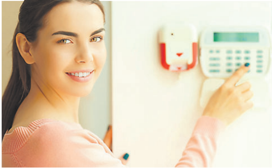
ALARM SYSTEMS: Many now even give remote camera access.
