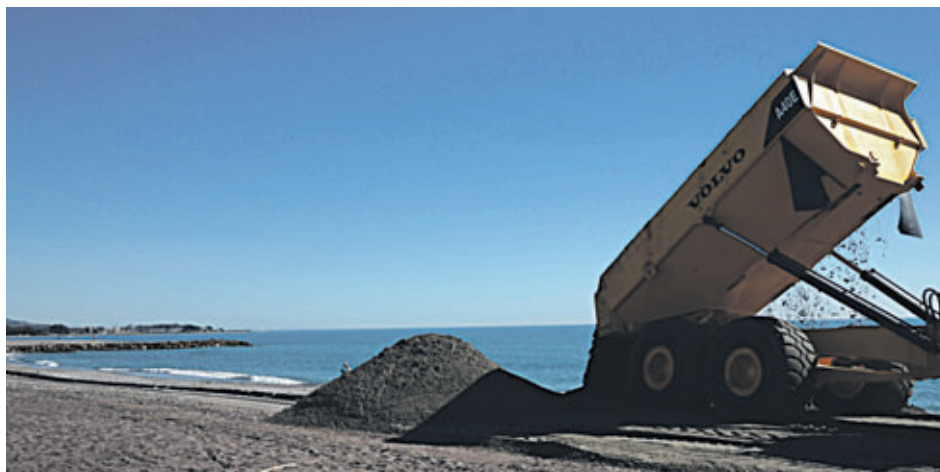
BEACH WORKS: Dozens of tons of sand will be brought in to make up for losses.
