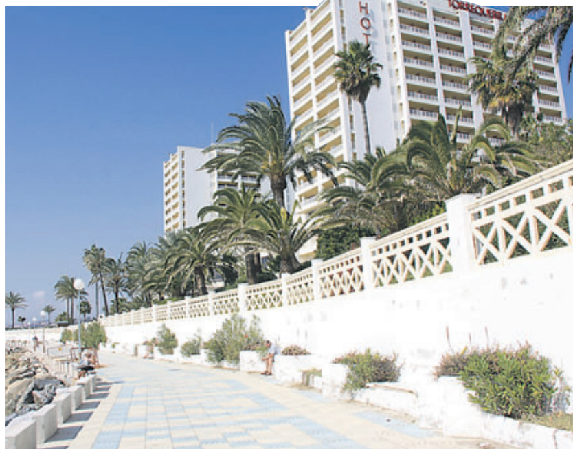
PROJECT RESUMED: Torrequebrada's Paseo will be ready for the summer.
