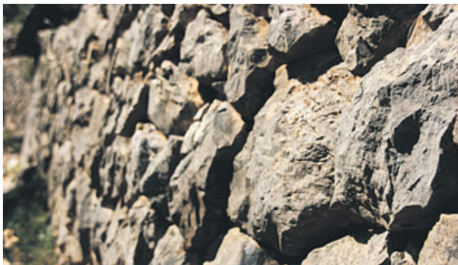
CULTURAL HERITAGE: Dry stone wall on the Ruta de Pedra en Seco hike.
