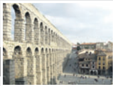
AQUEDUCT: 2,000 years old. |
