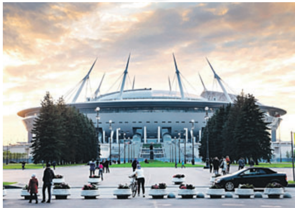
ZENIT: The new stadium still needs work before 2018.
