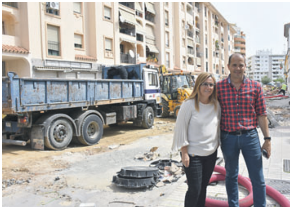
HEAVY LIFTING: Major roadworks in Fuengirola change downtown dynamic.
