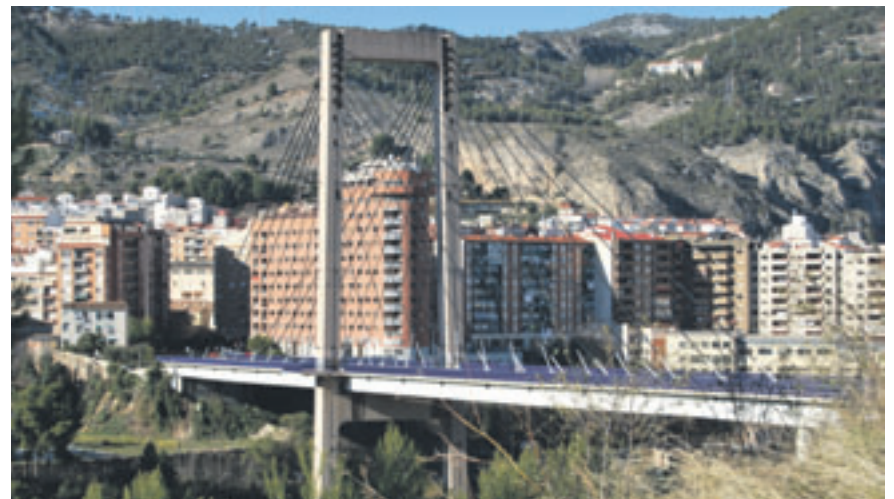
FERNANDO REIG BRIDGE: The cables are being replaced.
