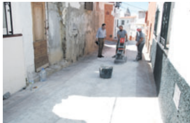
SMOOTH: Workers grind down the original road.
