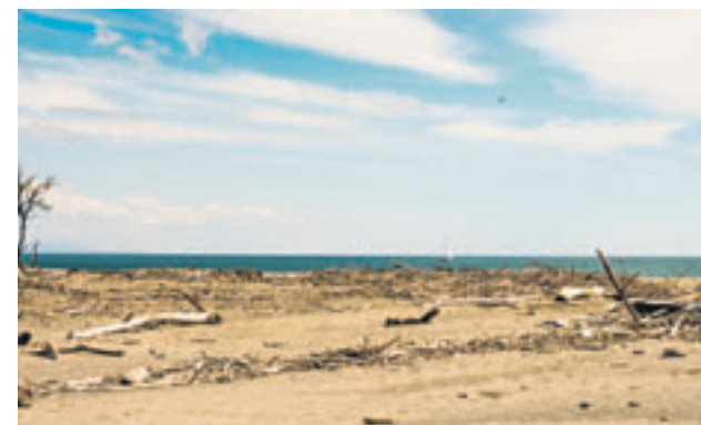
BEACH DAMAGE: Violent winds battered the coast.
