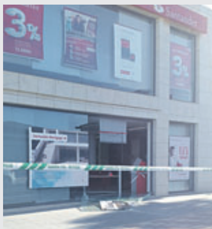
SHATTERED: Damage to the bank.
