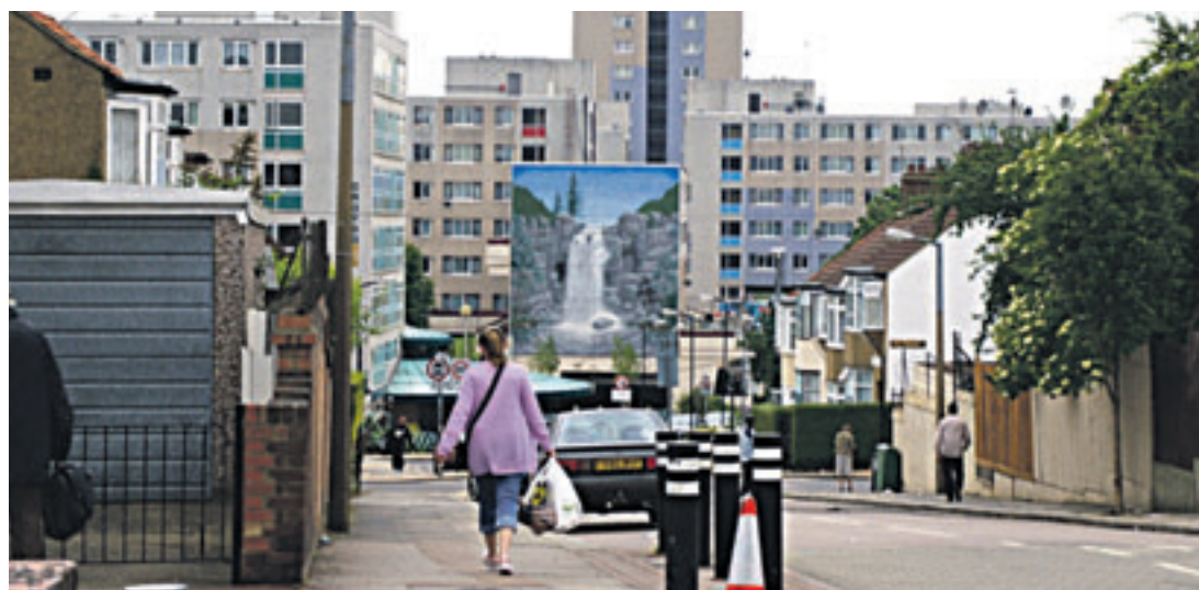
BROADWATER ESTATE: None of the buildings began their existence as slum dwellings.
