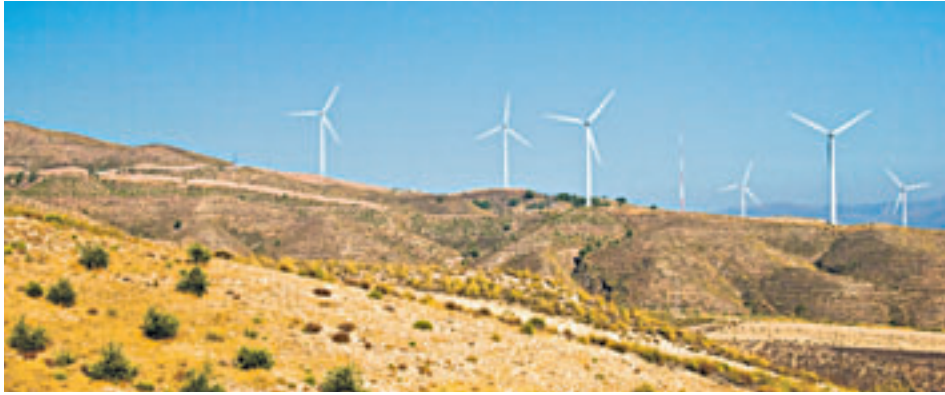
ELECTRICITY SUPPLY: The daily demand reached a historic level.
