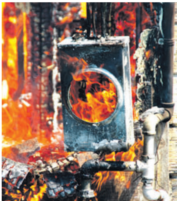
I SUMMER HAZARD: Air conditioning going full-blast.
