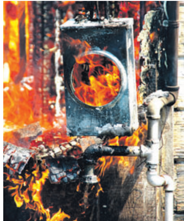
SUMMER HAZARD: Air conditioning going full-blast.
