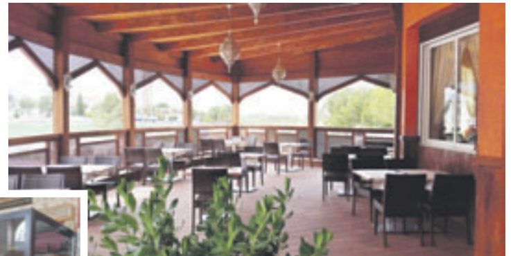
NEW LOOK: Attractive wooden terrace has been added.
