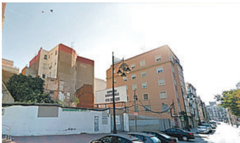
READY FOR EASTER: The site of the new hotel.
