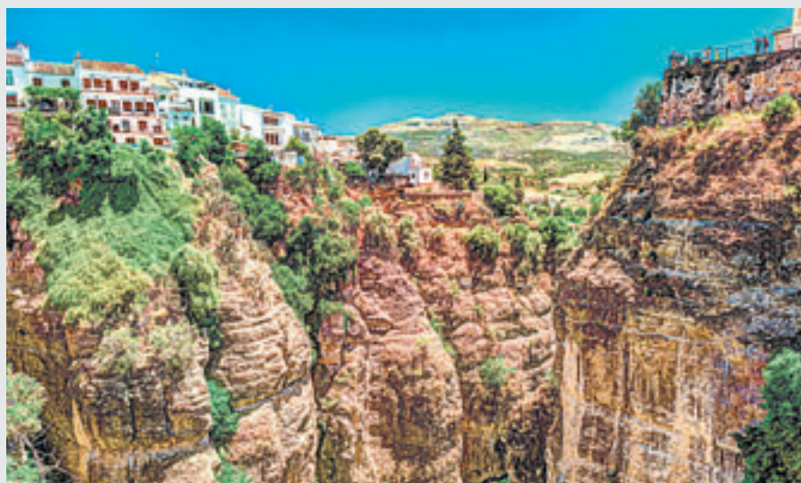
TAJO DE RONDA: Site of the new bridge.
