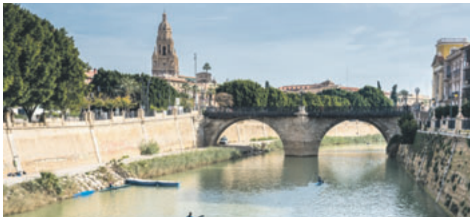
FOAMING: Test show pollution not behind River Segura issues.
