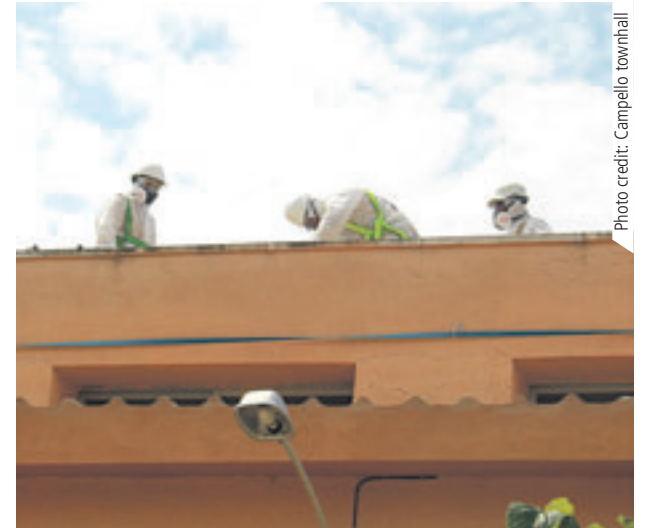
ASBESTOS REMOVAL: Hazmat suits for workmen at a Campello school last summer.
