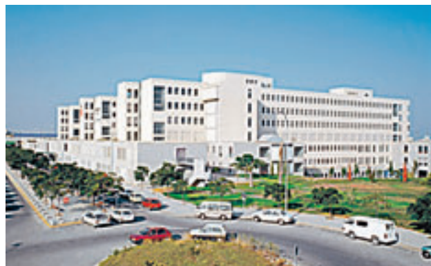
LIFT OFF: San Juan Hospital.
