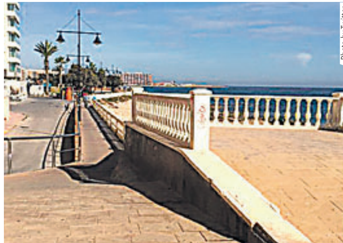
DELAYED: Work to begin next month or January at the latest.
