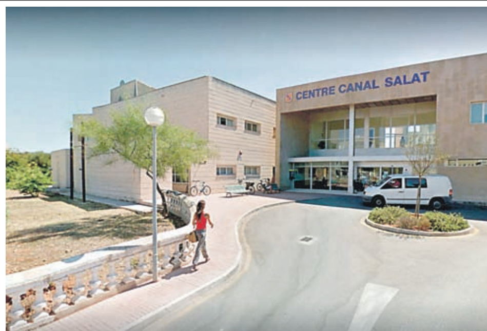
STEPS FROM HELP: The Canal Salat Health Centre where the incident occurred.
