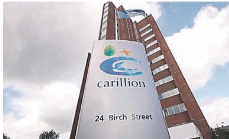
COLLAPSE OF CARILLION: Warning signs were there.
