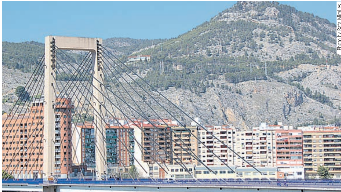
ALCOY BRIDGE: Cables have now been replaced.
