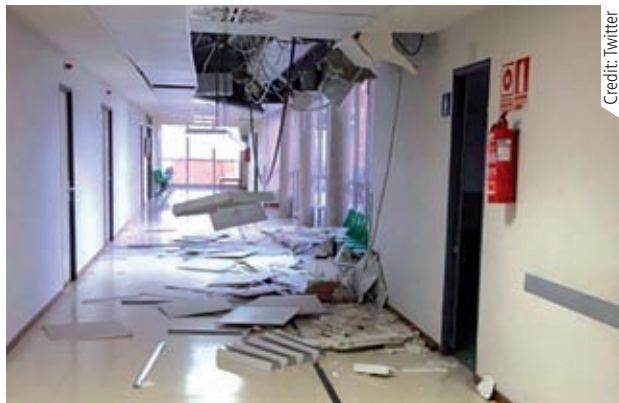
FALL: The corridor following the ceiling collapse.
