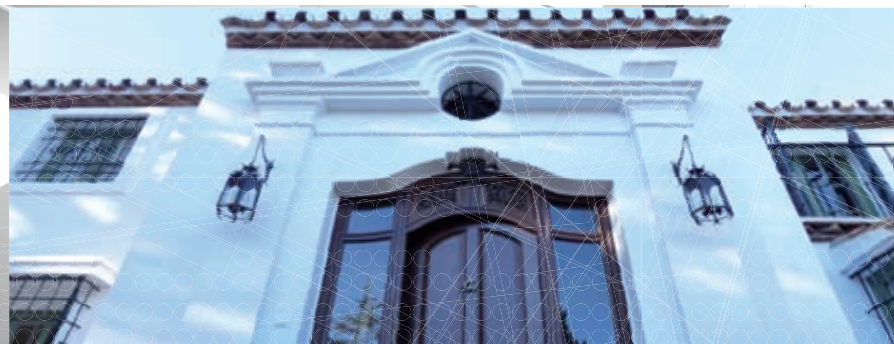
Entrance Refurbishment Benamara
