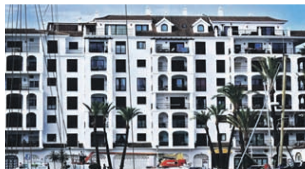
Renovation of Facades - Puerto de la Duquesa
