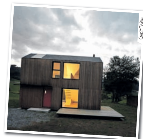
The house took just five hours to assemble on site.
