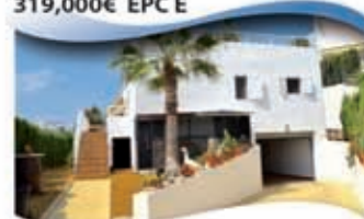
Ref: B1145 Located in Mojacar 319,000€ EPC E
