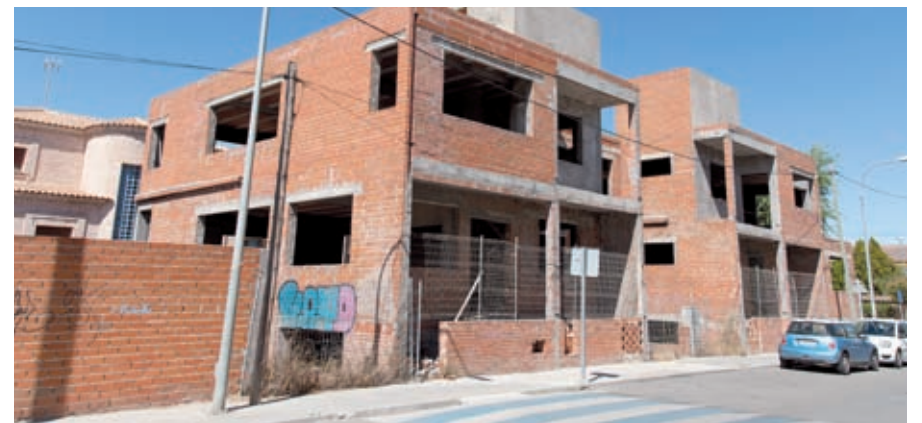
BUILDING BLOCK: The housing crash left Sesena littered with unfinished homes.
