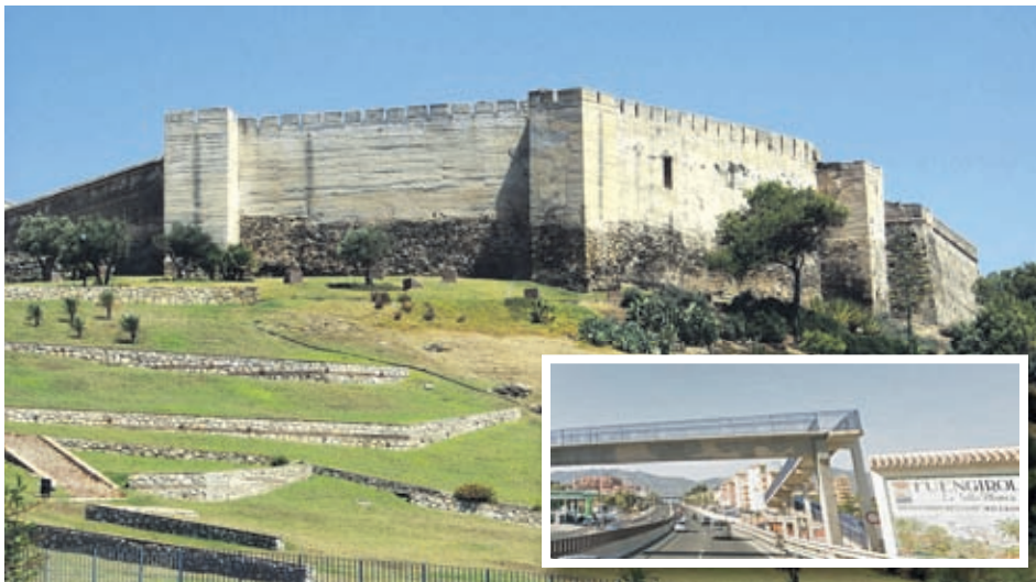
AT RISK: The bridge (inset) is near the Sohail Castle in Fuengirola.
