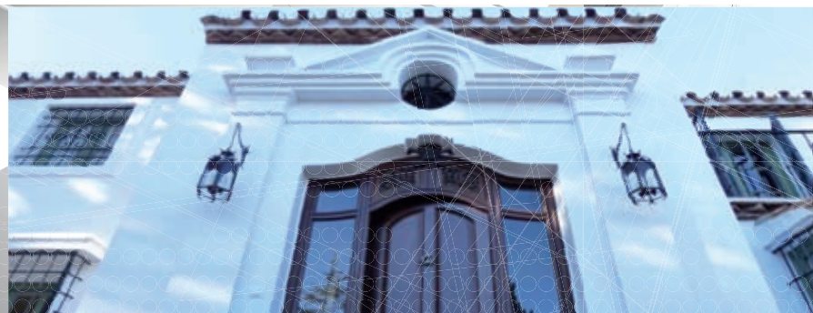
Entrance Refurbishment Benamara
