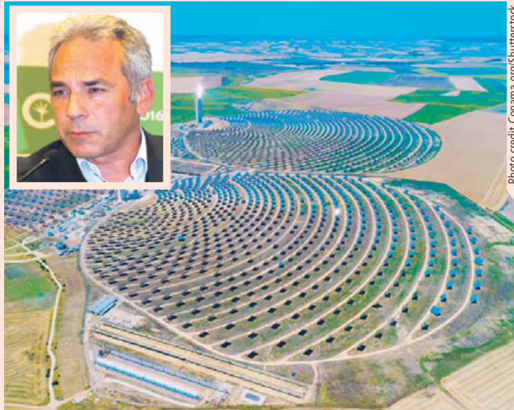
GOING GREEN: A solar energy plant in Sevilla and (inset) SGGG president Valentin Alfaya.
