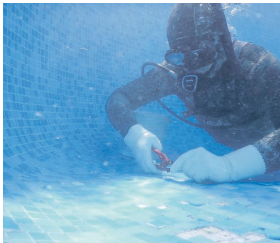
UNDERWATER REPAIRS: By a qualified diver.
