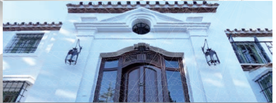
Entrance Refurbishment Benamara
