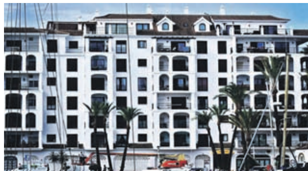
Renovation of Facades - Puerto de la Duquesa
