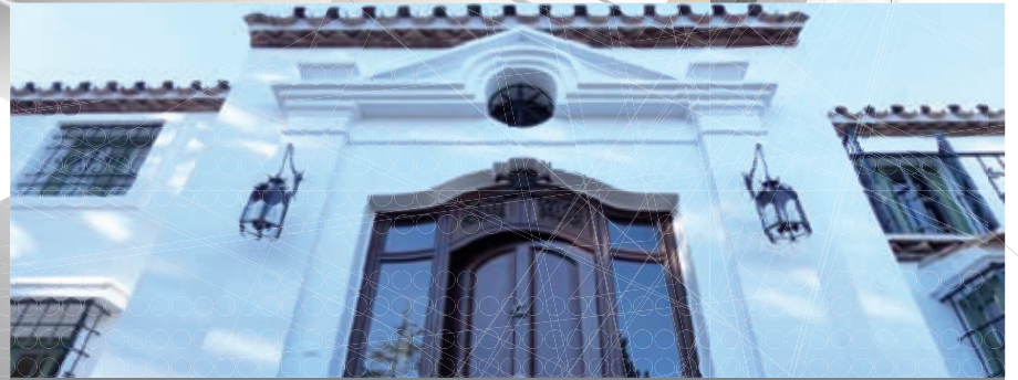
Entrance Refurbishment Benamara
