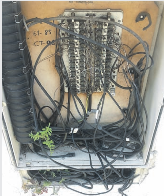
JUNCTION BOX: Open to the elements for three years.
